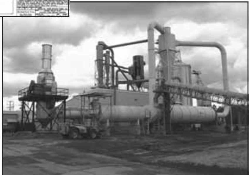
Completed 100,000 ton/yr Pellet Plant
